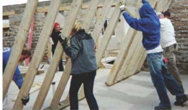
Blake High School volunteers raise an interior wall during spring break.
